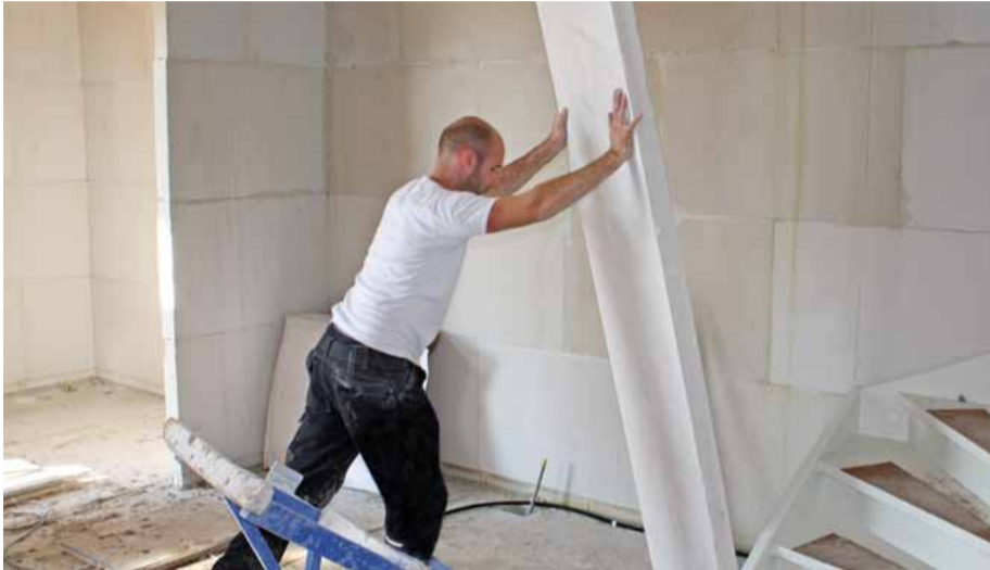
Ready for painting – super smooth panels do not require plastering
