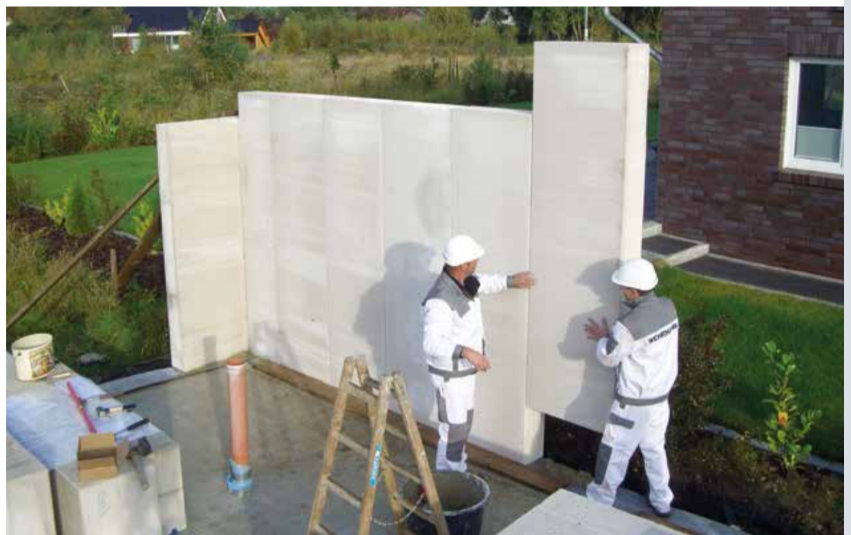
Vertical panels are highly suitable for fast building of standardised homes.
