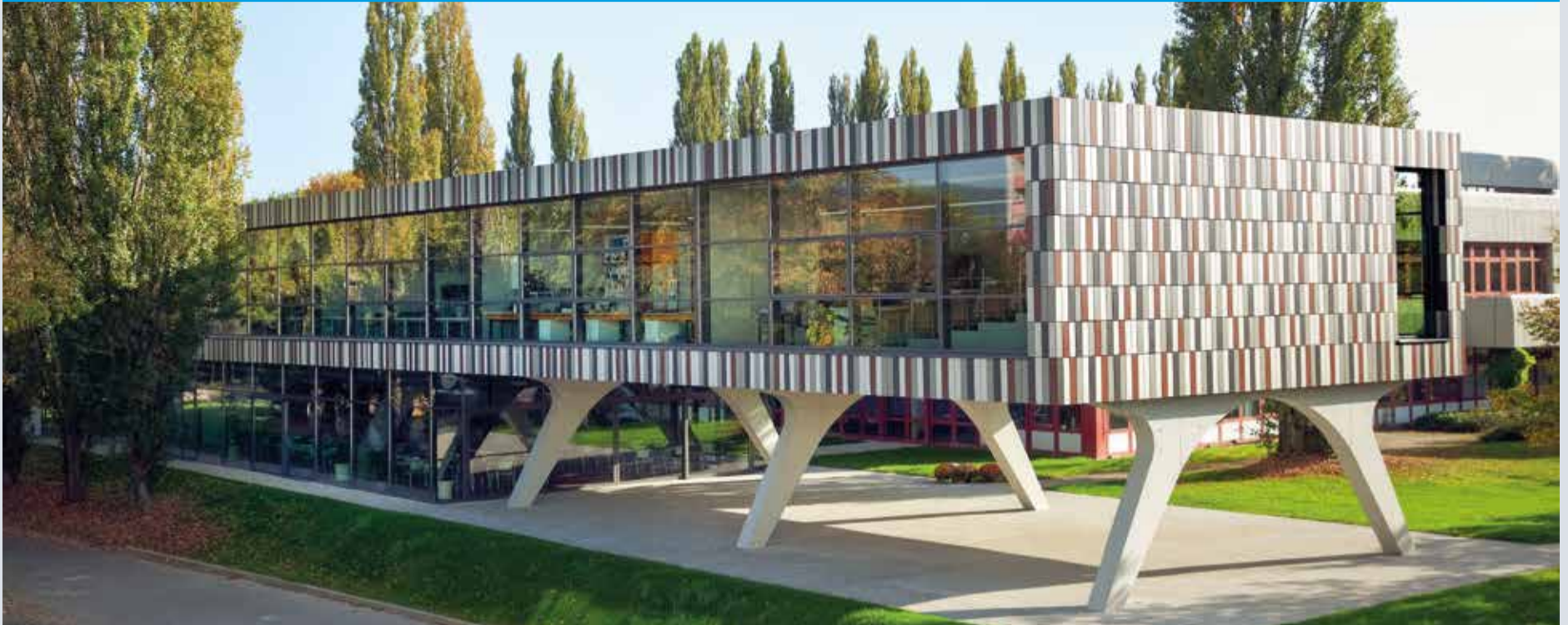
Architects love fibre cement sheets, elegantly finished with a wide range of colours or even unpainted, but coloured through with added pigments.
