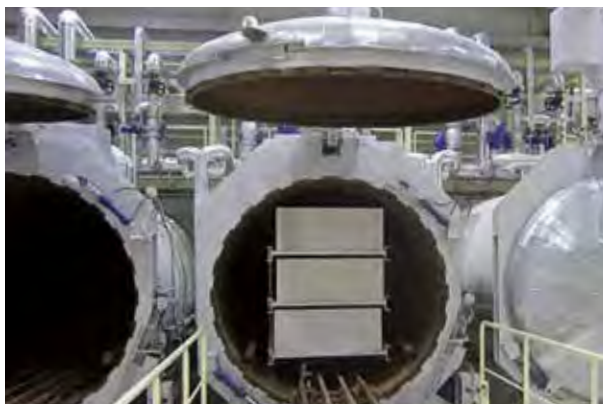
Autoclaving improves the material properties and contributes to sustainability
