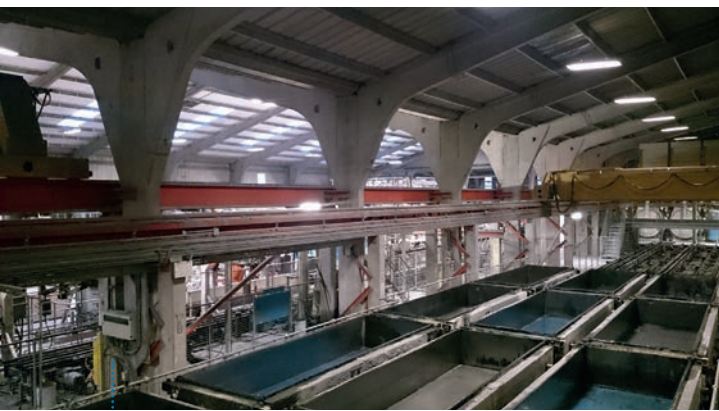
H+H Celcon before 2018: The old Wehrhahn plant is still producing good quality AAC, however the machines are no longer state-of-the-art.
