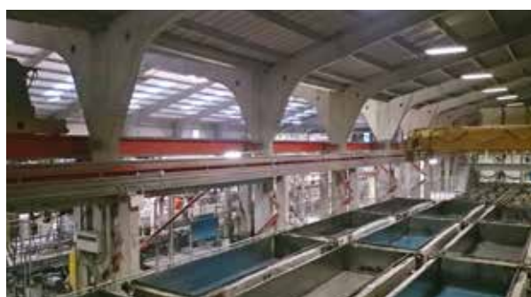
Before: Good quality AAC, however the machines were no longer state-of-the-art.
