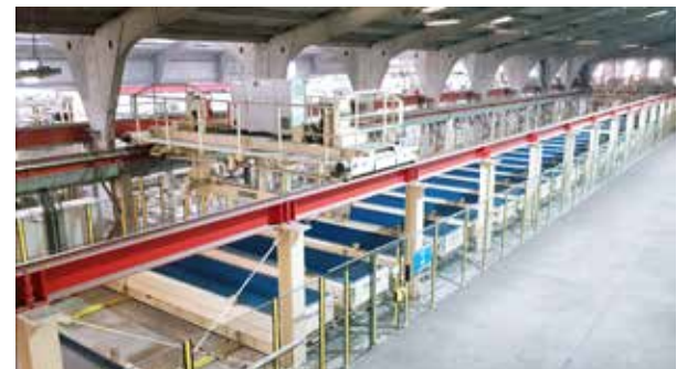
After: An impressive example of a full factory upgrade
