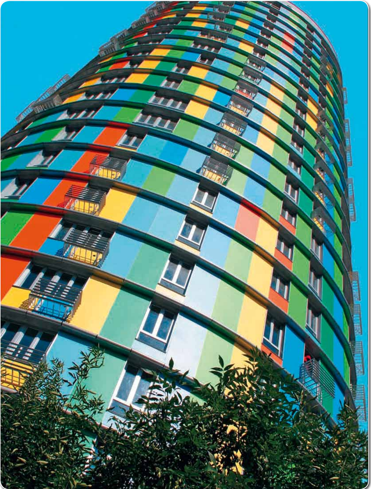
Colourful façades with highly compressed fibre cement sheets (Sheets have been produced by Minerit/Cembrit based on air-curing technology)
