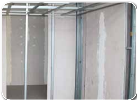
Dry walls on metal studs
