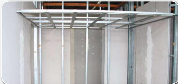
Dry walls on metal studs
